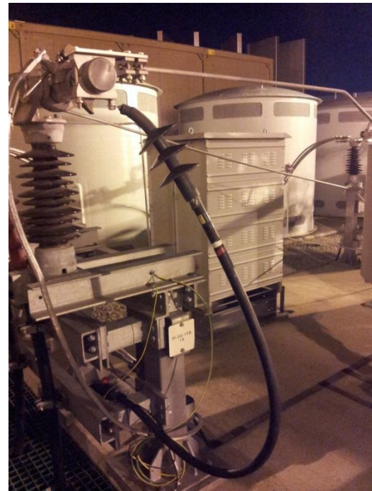
b) Voltage sensor measuring U_{b1} . The filter is connected to the open bus bar (see Figure 5-5a). The phase reactors and converter container can be seen in the background.
